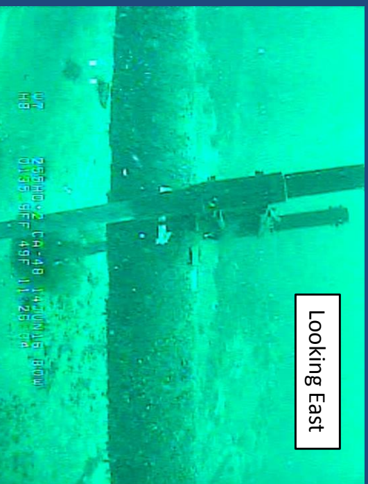
Laterally Deflected Anchor from 2016 Inspection
