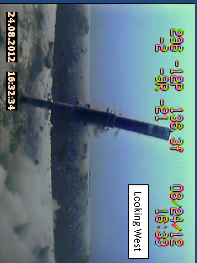
Laterally Deflected Anchor from 2012 Inspection
